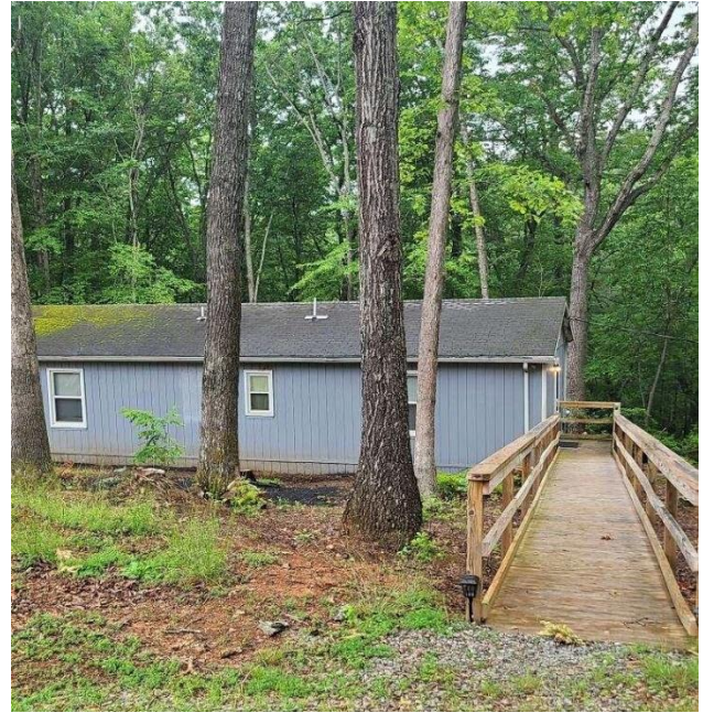
New ramp offers easier access to tribal cabin
